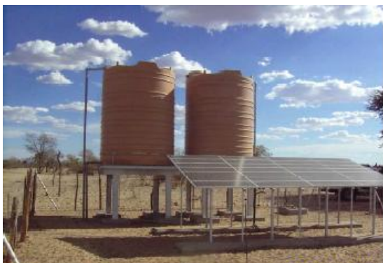
Figure 6.1: Small scale solar water pumping system (from: www.mme.gov.na )
